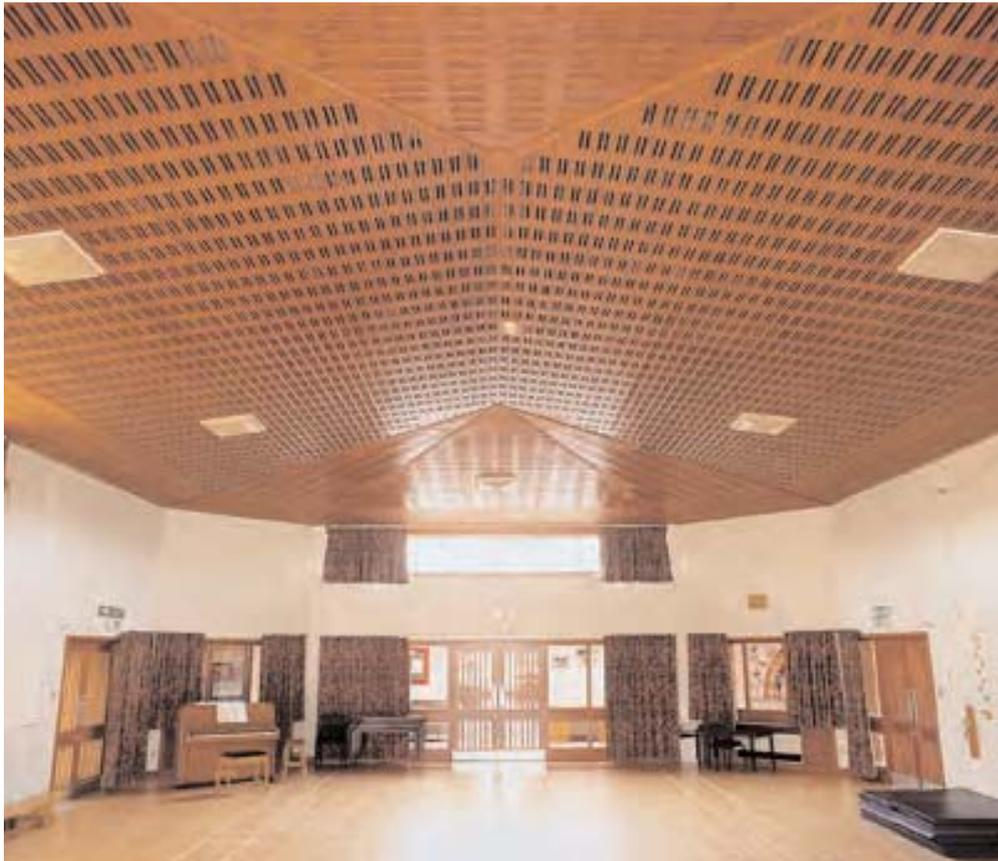
**Figure 7.1.3:** The hall ceiling after acoustic treatment
